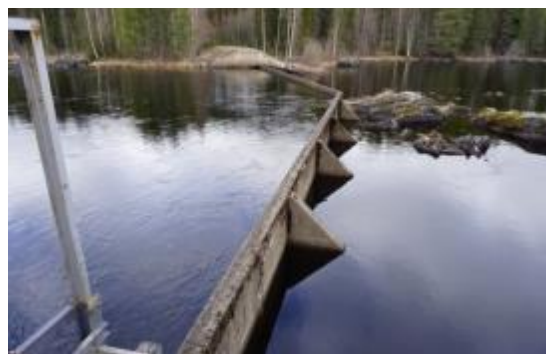
Dammvall i betong.
